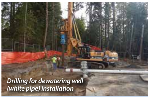
Drilling to install columns of sand and pea gravel around perimeter of wet well
