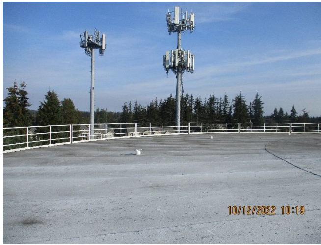
PHOTO 7 Cell Towers where Birds have Nesting
