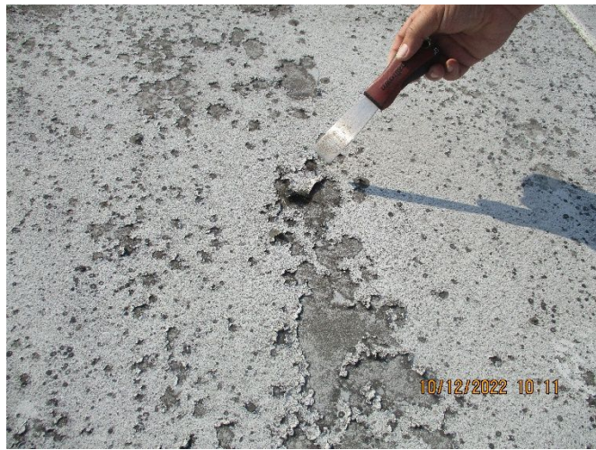
PHOTO 5 scapping off Topcoat
