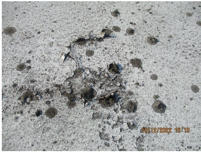
PHOTO 4 areas prior to scapping
